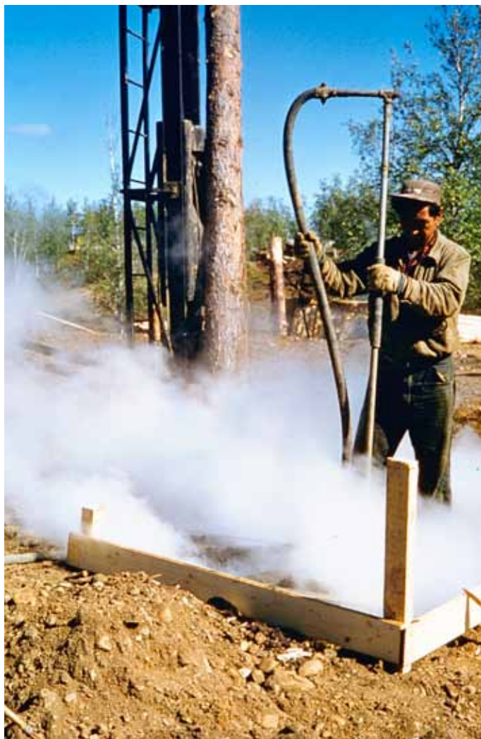
Sam Arey using a steam point to make a hole in the permafrost for a log pile, 1956. (Curtis L. Merrill/NWT Archives/N-1992-192-0199)
