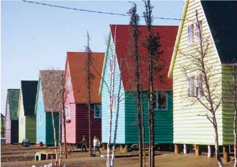
Buildings are erected on piles driven into the ground in order to prevent heat from the buildings melting the permafrost. (ICRC)
