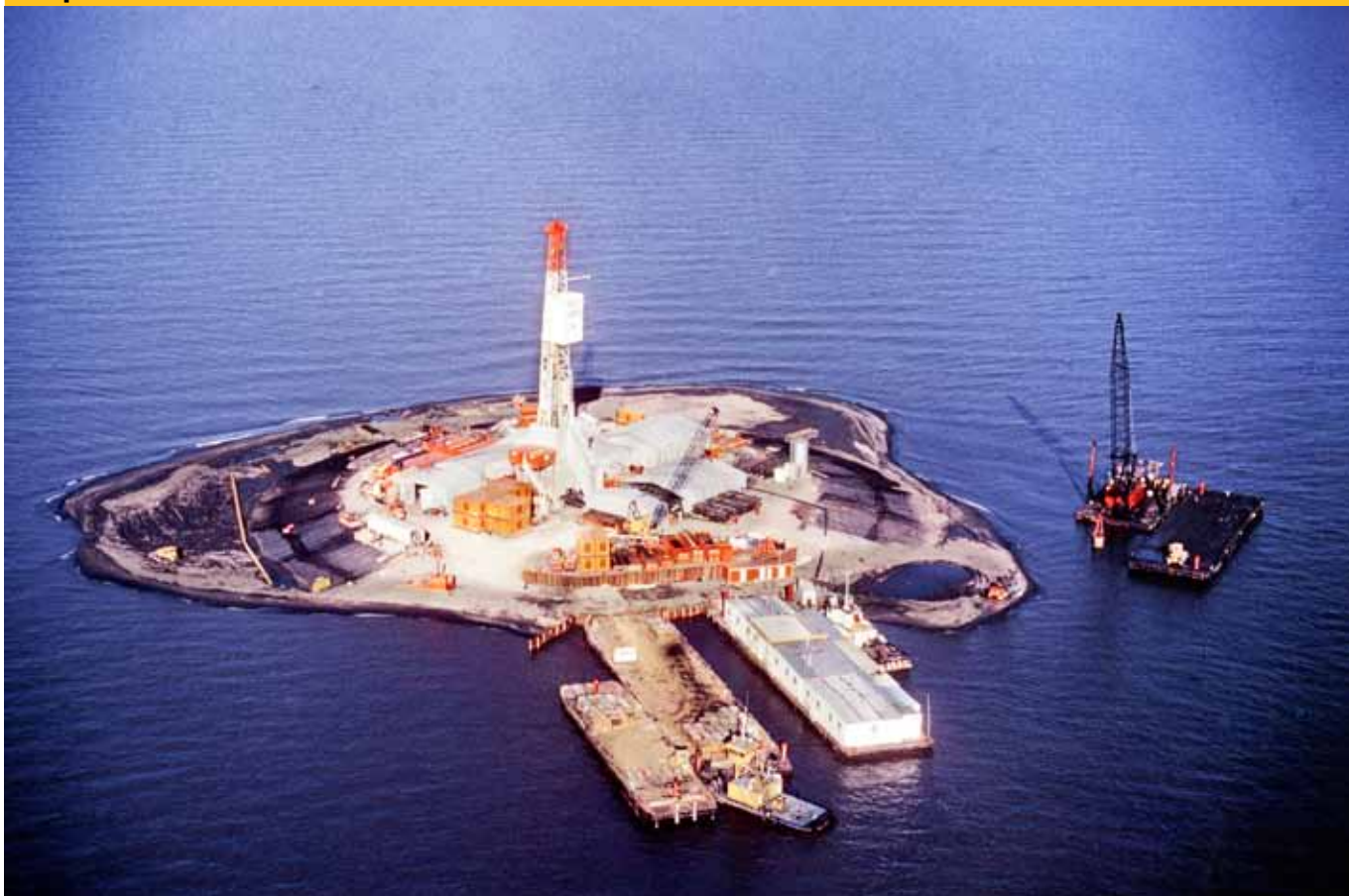
An artificial island facilitates drilling in the Beaufort Sea, 1973. (Imperial Oil Ltd./Glenbow Museum and Archives IP-14c-73-144)
